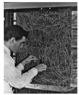
Frank Rosenblatt with the Mark 1 Perceptron Machine Perceptron Learning Algorithm (Linear Classification Model)
